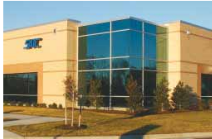
Science Applications International Corporation (SAIC), moved part of its Hampton Roads staff to this 23,000-square-foot office in Bridgeway Technology Center II to better serve its military customers.
