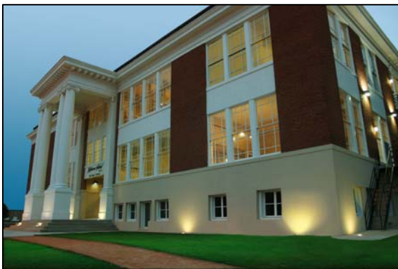
Jefferson School Lofts
