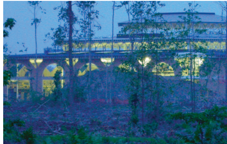
The new Lockheed Martin Global Vision Integration Center under construction.
